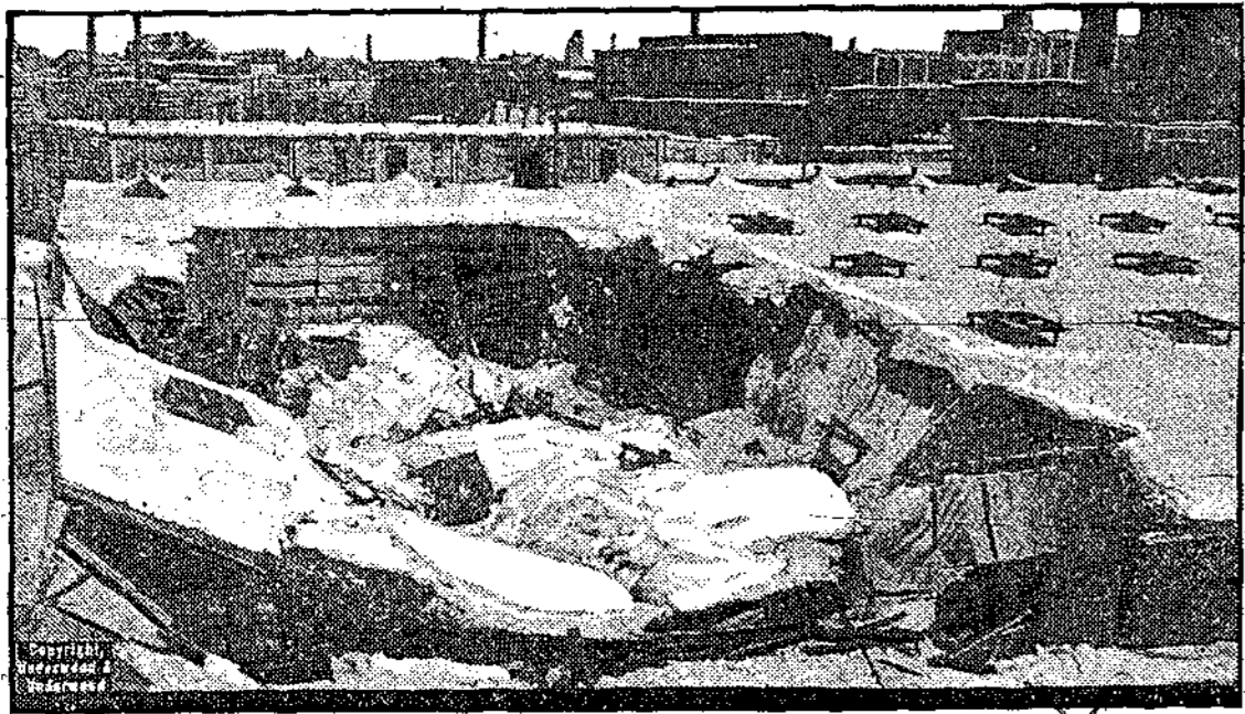
The severity of the winter in the East is indicated by this photograph. Weighted down by several thousand pounds of ice and snow, the roof of a storage building in Cambridge, Mass., recently collapsed, completely demolishing the structure. Luckily no one was inside when the accident occurred.
