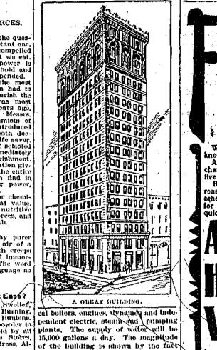
that there will be about 2,000 electric Hee where a road onds before you lights, 50,000 feet of electric wiring, seventeen miles of piping, and the weight of the steel frame work will be about 2,000 tons.
