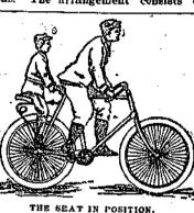
spring-constructed braces connected to the rear uprights of an ordinary diamond frame bleycle. It extends downward and connects with the frame by properly constructed clips. At the top it is connected to the frame by an ingenious clamping contrien both steady and strong, and is further secured in place by cross clips and thumb screws. The braces being bent sultably insures a spring seat, The contrivance can be attached to any bicycle in a moment, and be re-
